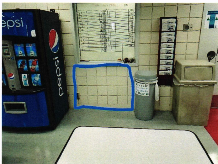
Unit 9100 charging cart location. Existing power may be sufficient.
