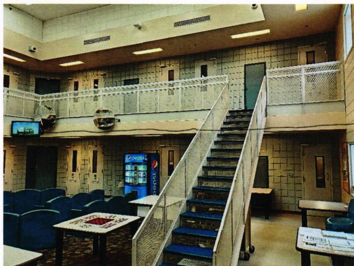
Unit 3100 first part of conduit run to WAP location.
